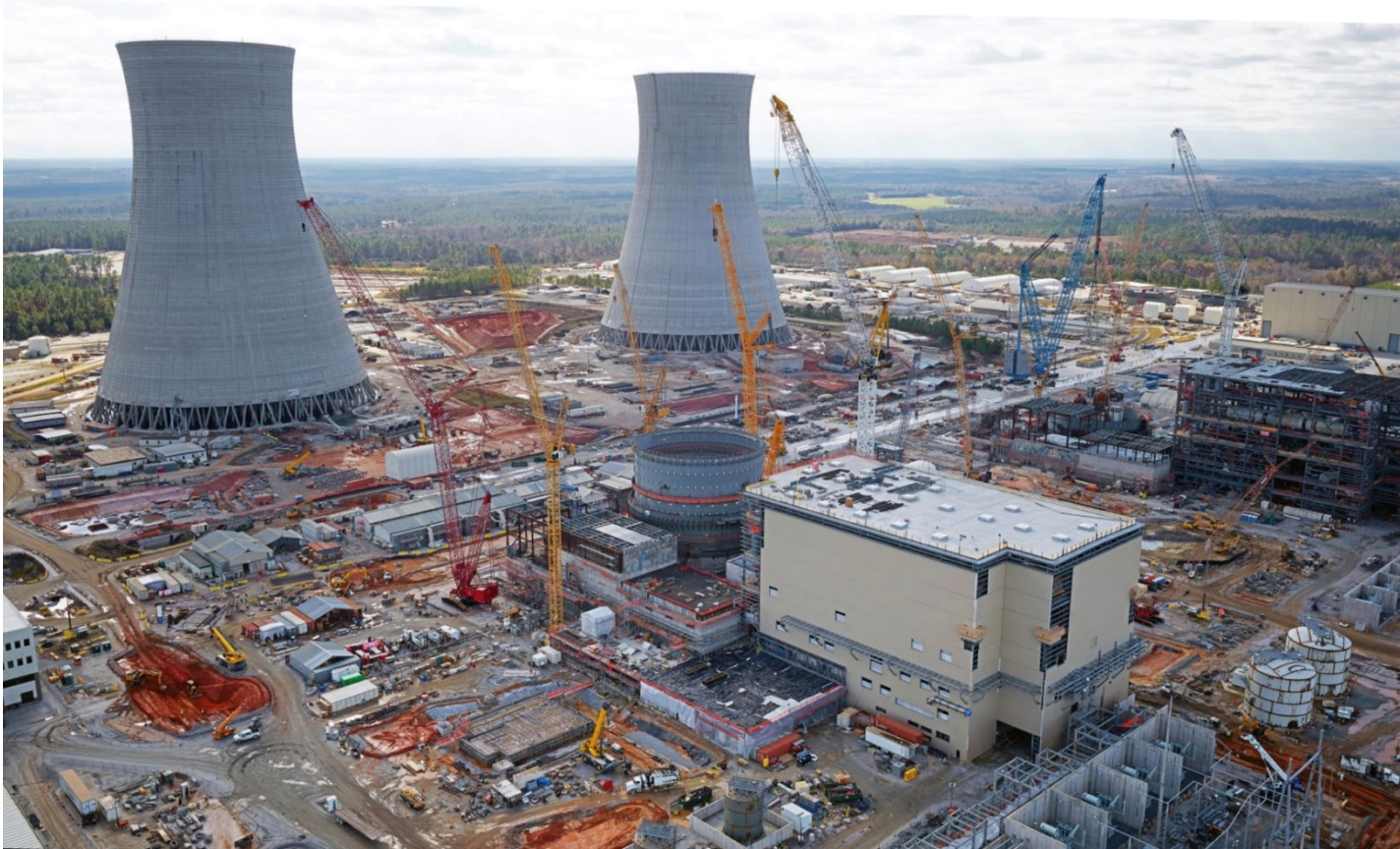
Vogtle 3 and 4 Site
