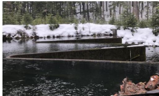
Stone Creek Hydroelectric Project (12 MW)
