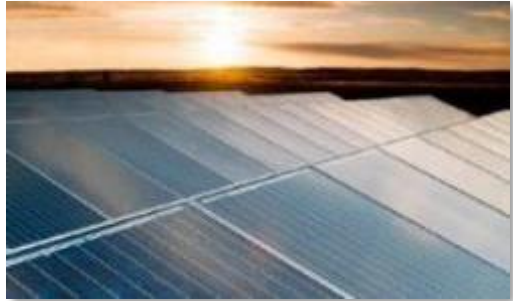
White Bluffs Solar Station (38 KW)
