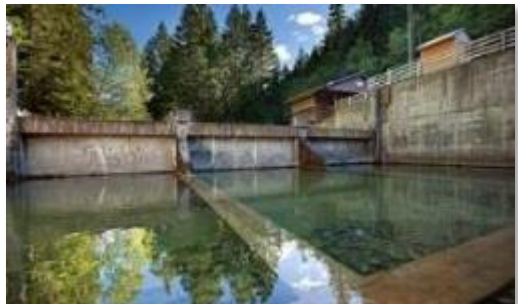
Packwood Lake Hydroelectric Project (27 MW)
