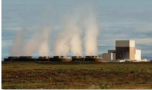
Columbia Generating Station (1,207 MW)
