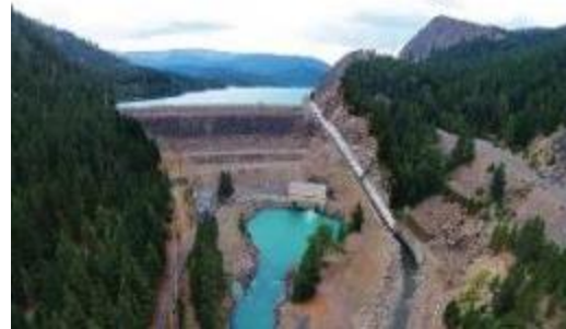
Tieton Hydroelectric Project (15 MW)
